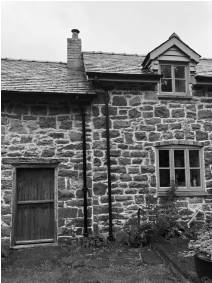
PLATE 3 The re-built cottage abutting the mill
