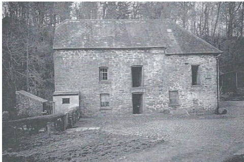
PLATE 10 The south-east face (Note: the join is on the right hand edge of the two doors, not on the roof line change: the wall-plate from the original building can be seen below the later roof)
