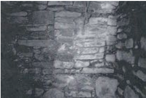
PLATE 22 The blocked window indicates that this was once an outside wall
