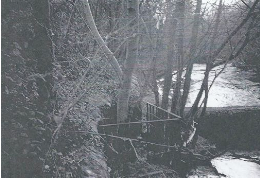
PLATE 8 Struet Mill intake behind railings
