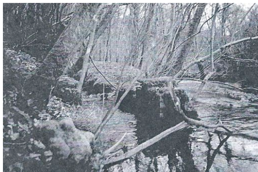
PLATE 25 The stone abutments of the sluice leading to the leat, with slots for the gate evident in the stone
