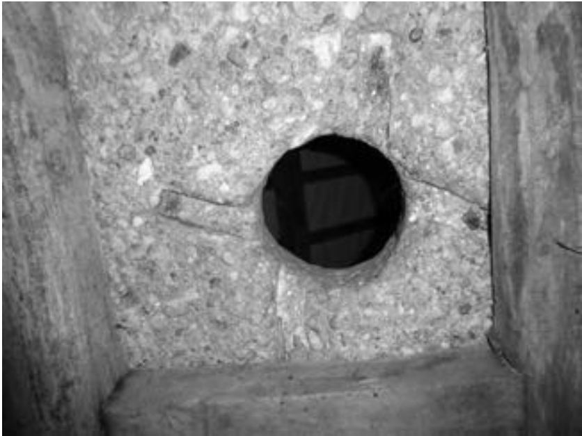
PLATE 11 The upstream runner stone from below showing rynd recess
