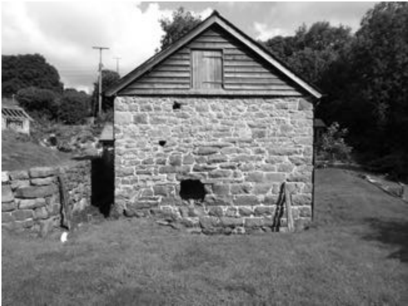
PLATE 1 The end wall, showing the shaft-hole for the waterwheel and positions of the trough support and water control to the wheel
