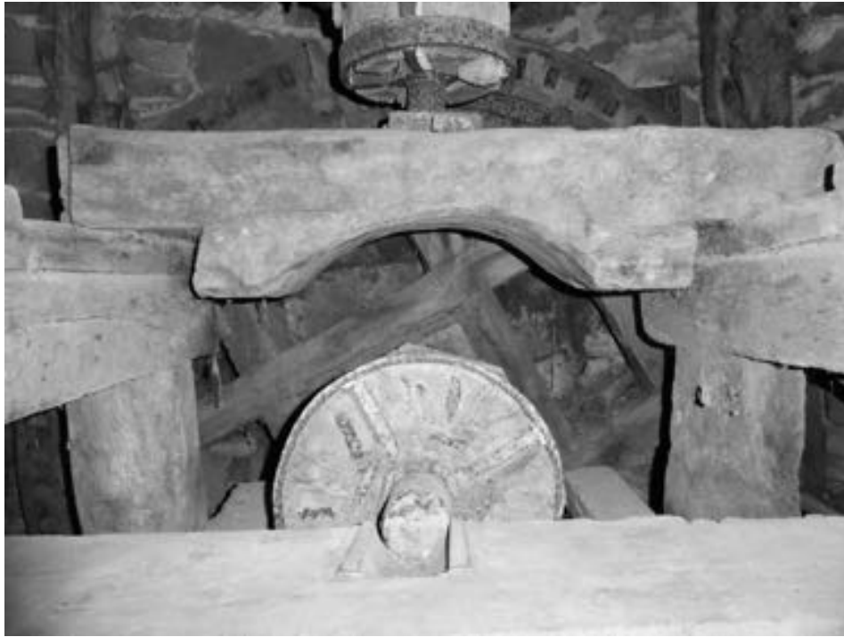
PLATE 4 The inner bearing of the wheel-shaft with the sprattle beam supporting the upright shaft
