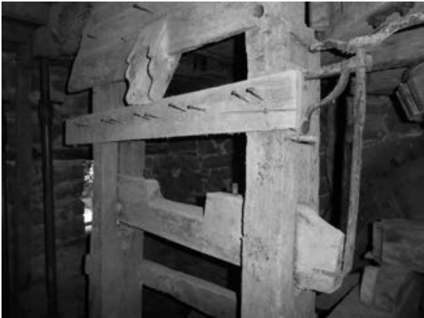
PLATE 9 The front bridge-posts of the downstream pair of stones with brayer and tentering control
