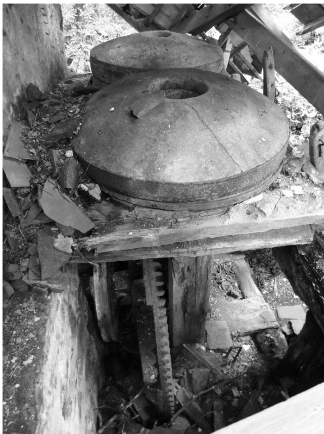
PLATE 2 Machinery in the collapsed Melin Trygarn
