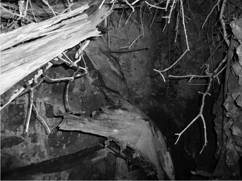
PLATE 1 Wooden Shrouds from the Wheel at Melin Bodwrdda
