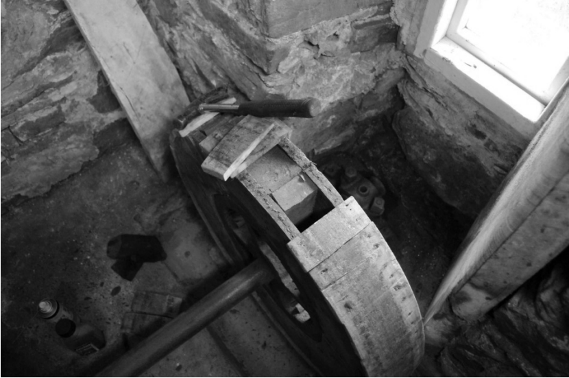
PLATE 1 Repairs to rim of lower pulley
