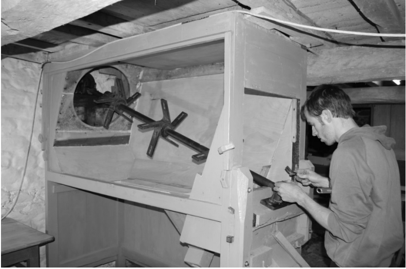
PLATE 6 Repairs to the interior
