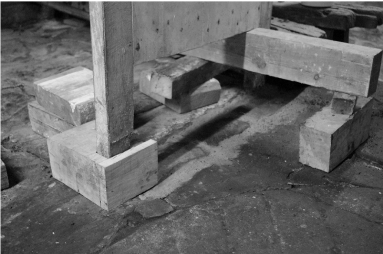
PLATE 3 Repairs to oak support in progress
