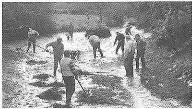
Clearing Weeds in Empty Pond
