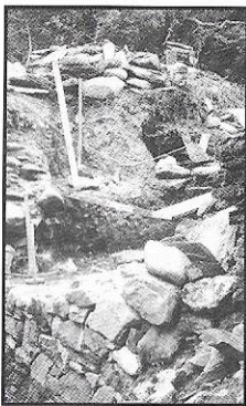
Dam being repaired
