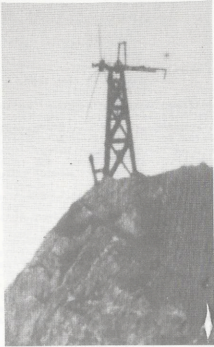
10. The derelict windpump
