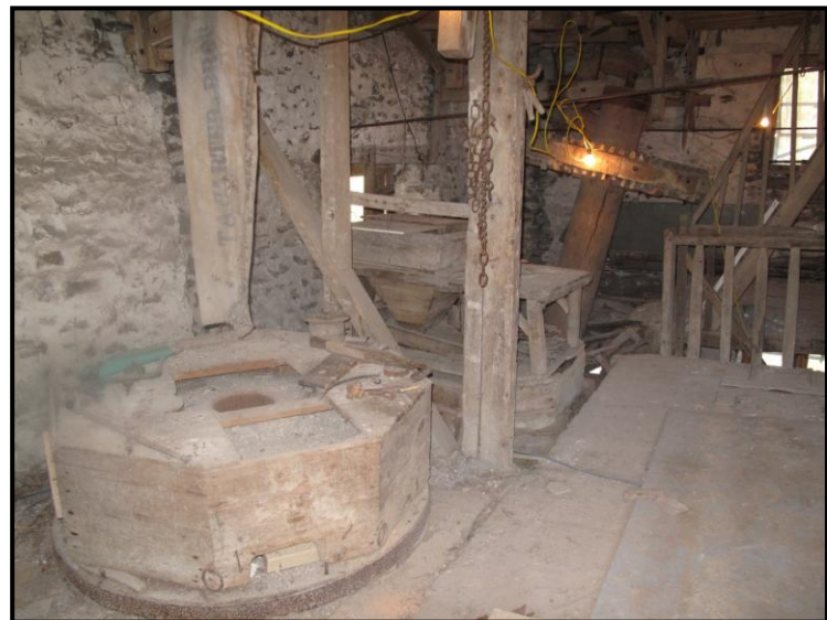
Melin-y-ddôl stone floor showing the displaced main shaft and spur wheel
