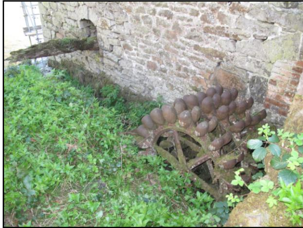
Melin-y-ddol: remains of the waterwheel axle and the three-gang turbine
